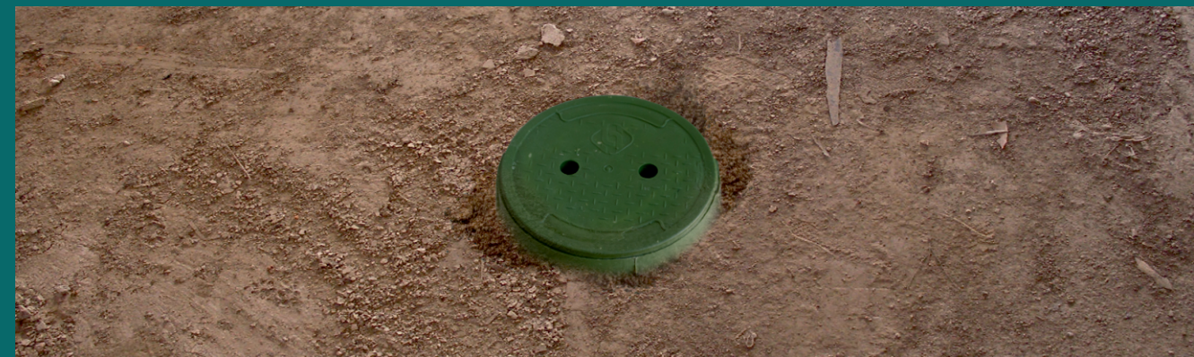
Step 6. Cover the TruePower Earthpit Cover with soil and ram properly
